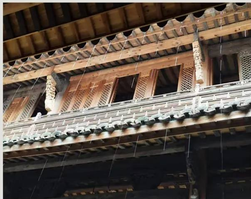
03 檐下实景 UNDER THE EAVES
