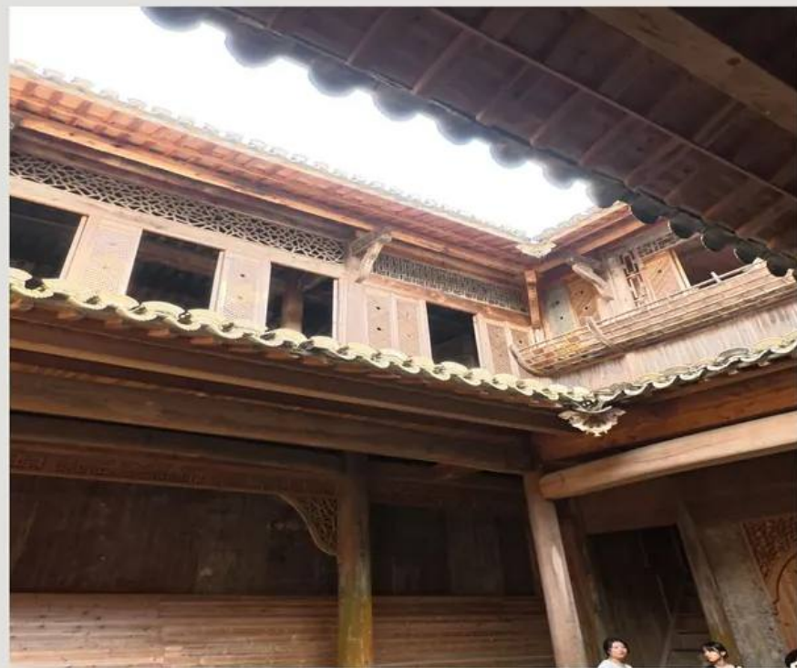
02 天井仰视 COURTYARD / LOOKING UP
